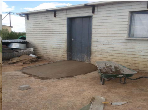
Pic 2: Building of wheel-chair ramp
